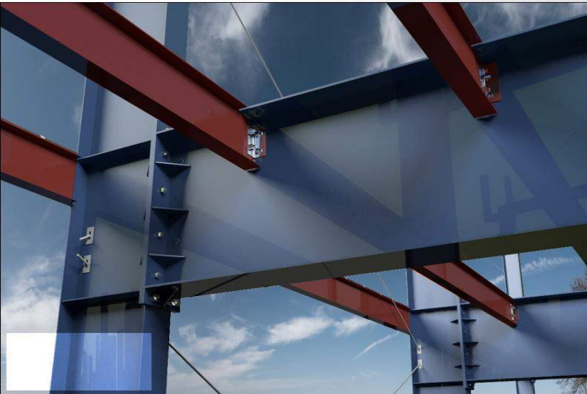
BEAM-JOIST CONNECTIONS
